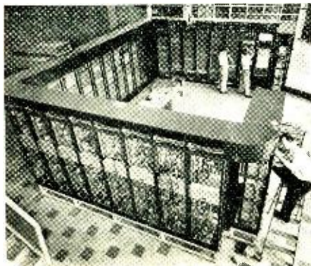
Workmen are placing building-block units in the 31 vertical channels of UDEC II .
